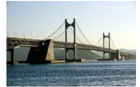
Gwangan Bridge in Korea
